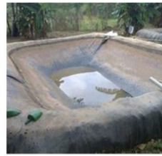
Excavated pond with liner
