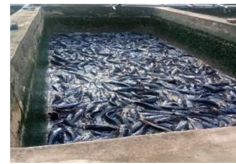
A concrete tank for raising catfish
