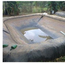
Excavated pond with liner
