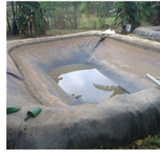
Excavated pond with liner
