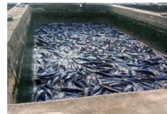
A concrete tank for raising catfish
