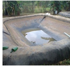
Excavated pond with liner
