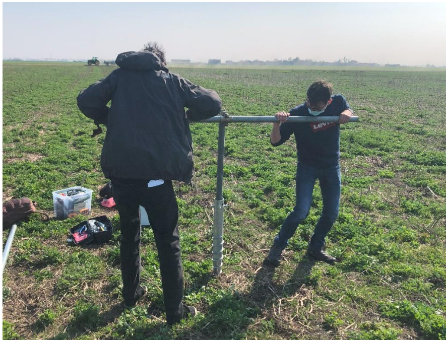
Figure 3 installation of the screw foundation
